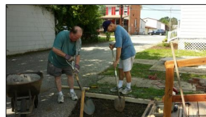
Bruce Grine (L) and Bob Greenwalt installing the concrete ramp pad.
